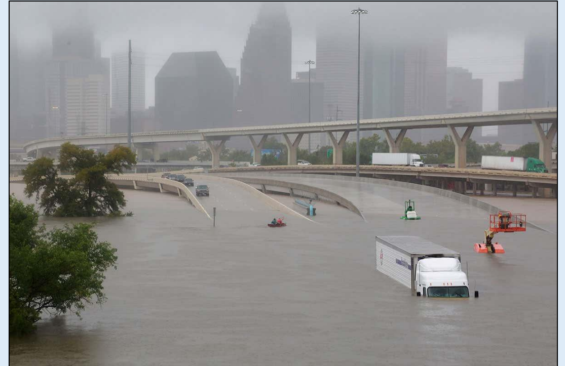
Flooding following Hurricane Harvey in Houston, TX
